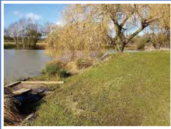
Man-made concrete inlet to pond
