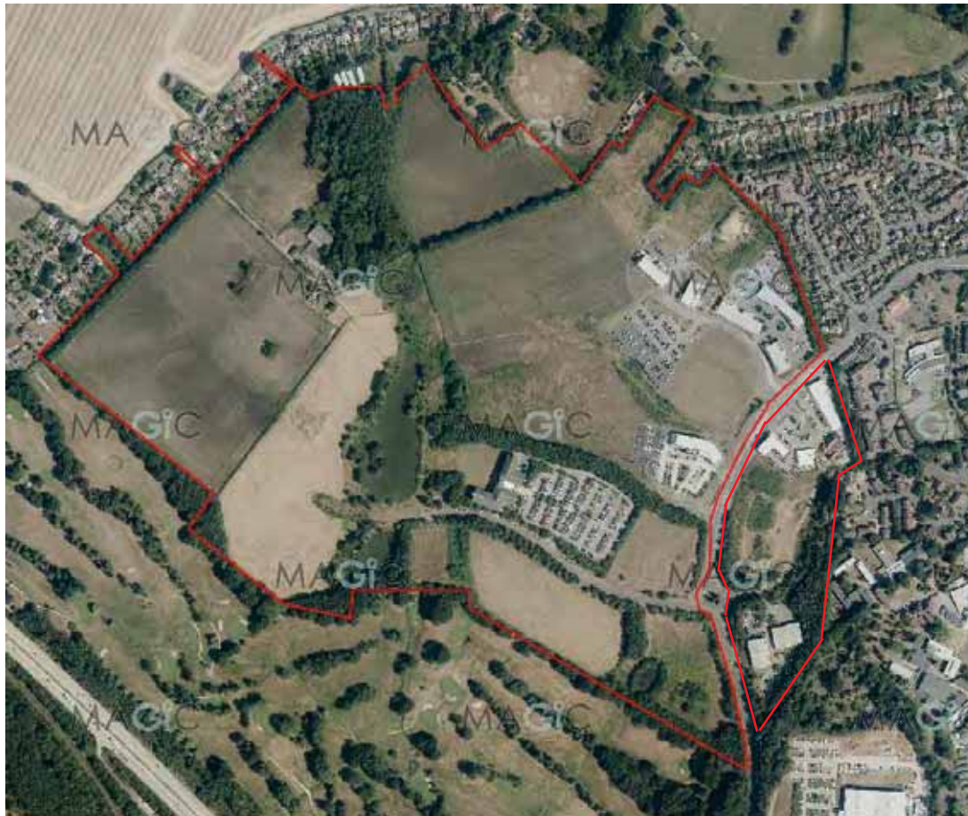
Figure 1.2: Aerial view of the proposed development site (red line indicative).
